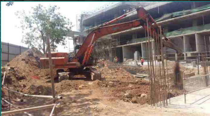
Backfilling
